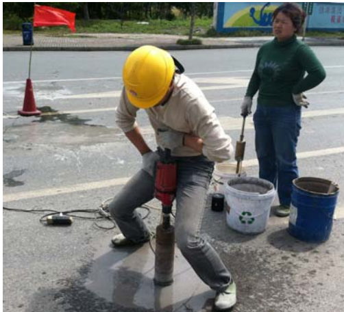
Figure13 Drill holes
