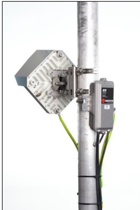
Figure 26 - Surge Arrester fitted to pole
