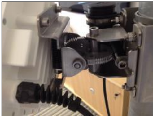
Figure 17 - Alignment bracket
