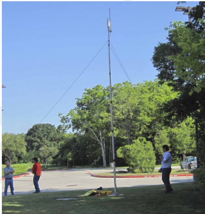
Figure 3-31 Backhaul Antenna Erected
