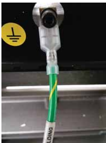
Figure 4-118 Ground wire connected to panel
