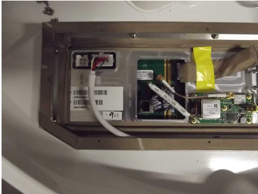
MIM, SSM and EGR of primary antenna installed
