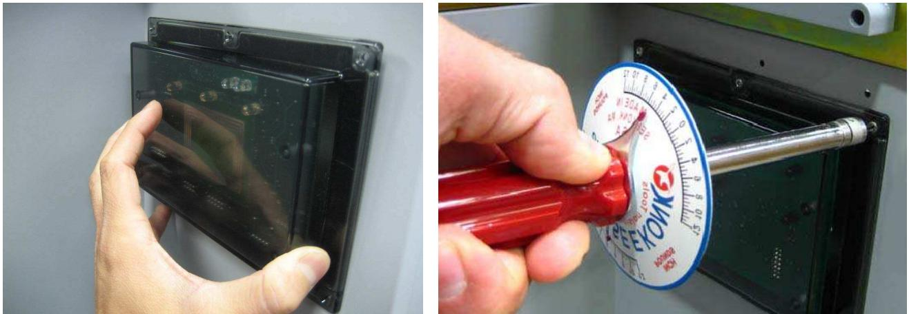
Locate Assembly, Window/PCB RFID/Software in opening of Weldment, Bay and secure with 6 Screw, Oval Head, Phillips, #4-40 X 5/16 (31-298-001). Torque to 6 in-lbs using torque driver and #1 phillips bit.
