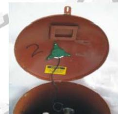
B.) **REMOVE** the ON/OFF magnet from the bottom of the propane transmitter to turn the unit on and apply extra bar code to customer paperwork.
