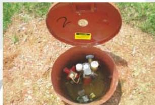
**REQUIREMENT:** Propane gauge must be a **Remote Ready Gauge**. See gauge kit 0004264 for adapting a non-remote ready gauge
