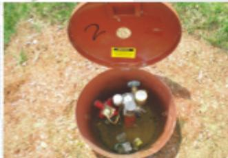
**REQUIREMENT:** Propane gauge must be a **Remote Ready Gauge**. See gauge kit 0004264 for adapting a non-remote ready gauge
