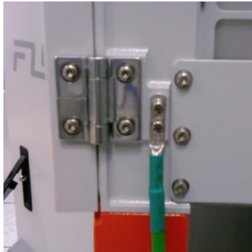
[Figure III-24 Ground cable connection drawing]
