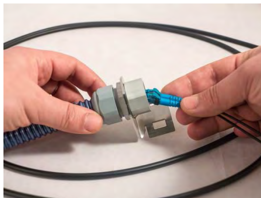
4 Push FO cable from LC connector side through the conduit.
