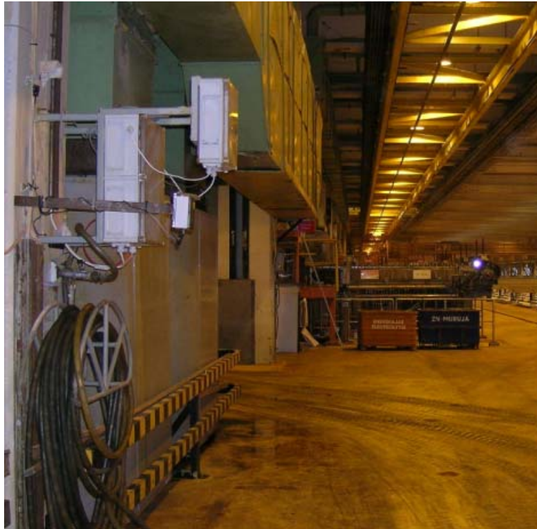
Figure 7. Gateway Device (smallest box) mounted on the wall of a cell house.
