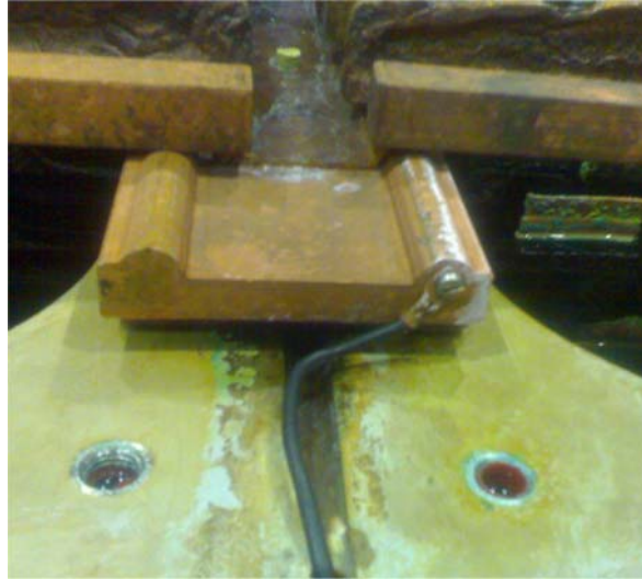
Figure 13. Bus Bar Tap with Screw.
