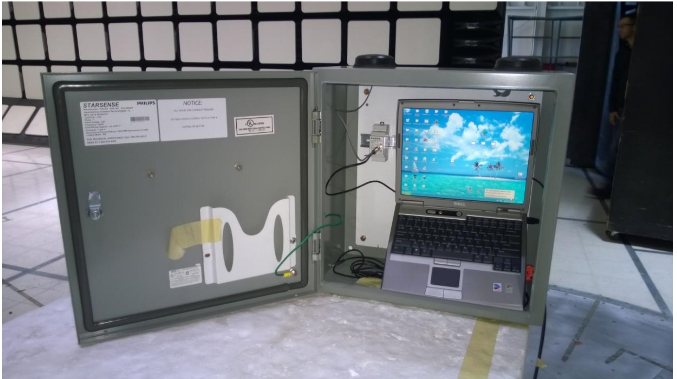
Figure 27 – View inside the cabinet
