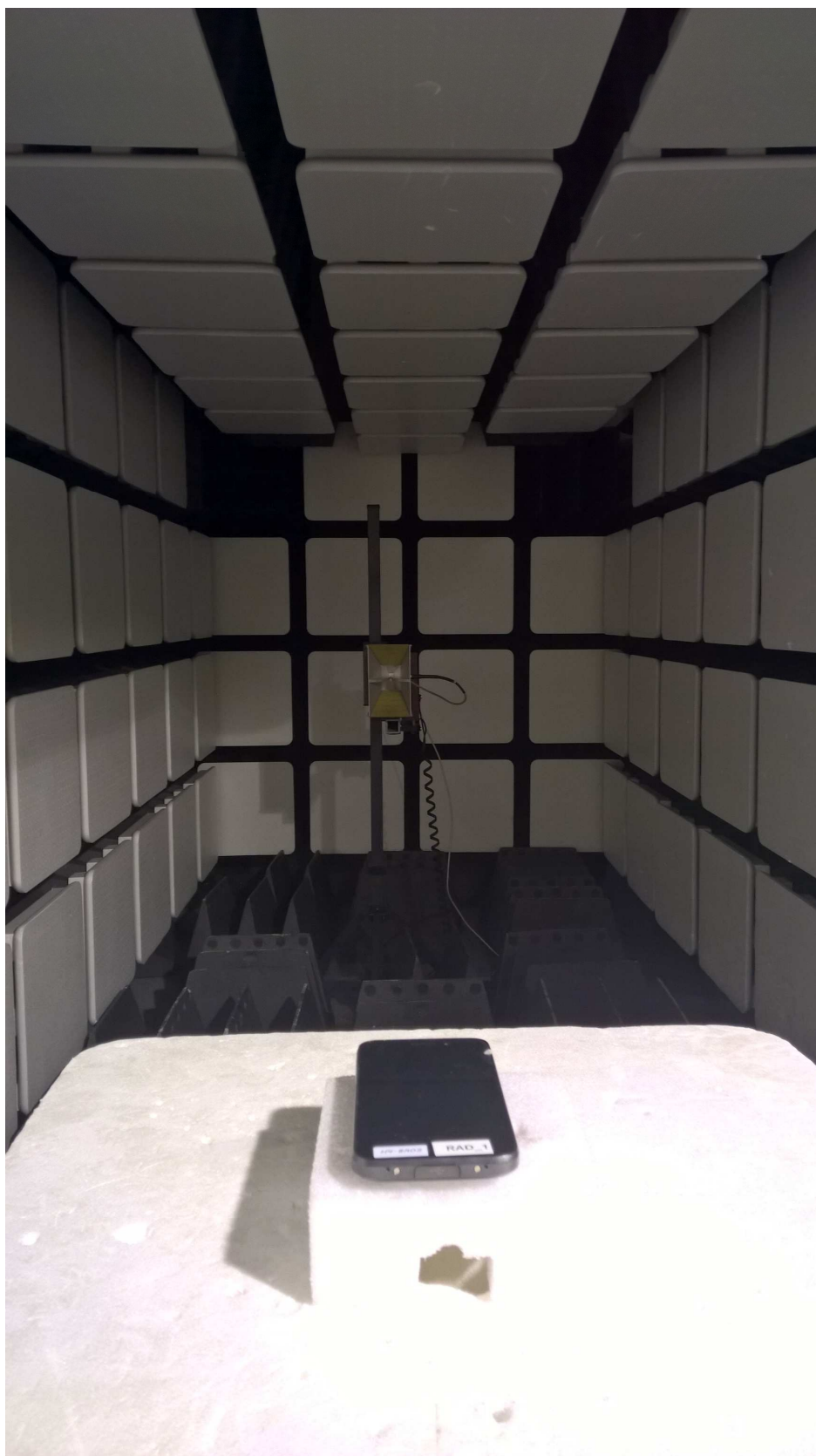
Radiated test setup 1 – 18 GHz, EUT horizontal
