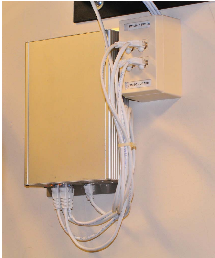
Fig 5 – Finished Collector installation with Remote Radio terminal block.
