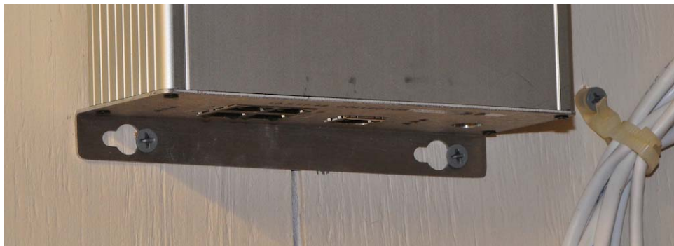
Figure 7: Collector on mounting screws after tightening.
