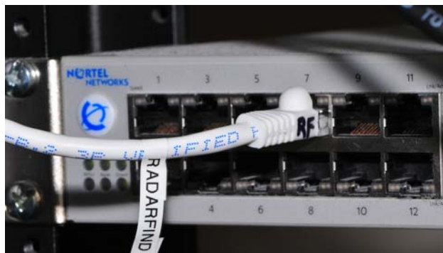
Figure 10: Collector Ethernet jumper clearly marked at switch end.
