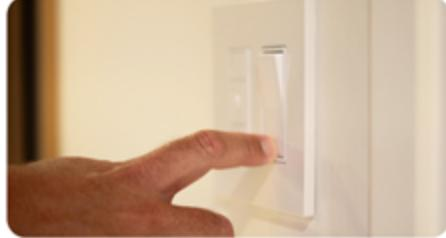
Before installing your camera, locate the power switch for the light fixture where you wish to install, and turn off the power.
