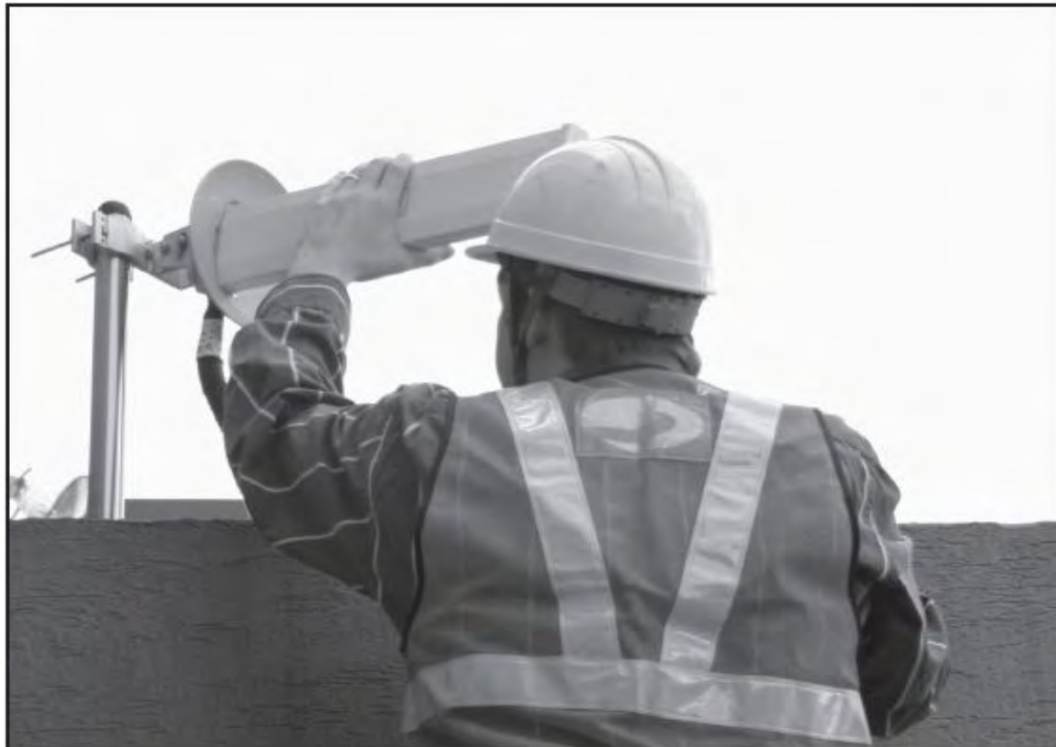
<Figure 4> An installer is directing Donor Antenna to nearby BTS to receive strong input signal.
