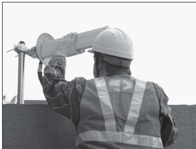
<Figure 4> An installer is directing Donor Antenna to nearby BTS to receive strong input signal.
