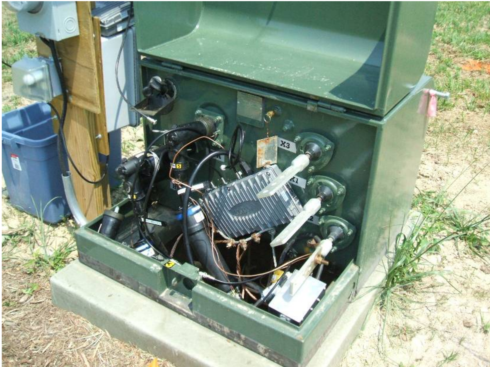
Photograph B-8: Test Site Photo – CURRENT Technologies Field Research and Test Area - XFMR X3 - Interior view, MV1 Bridge
