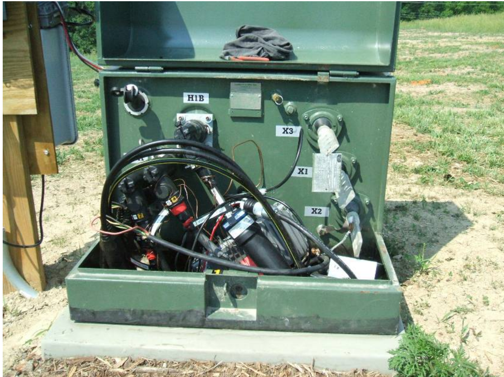
Photograph B-5: Test Site Photo – CURRENT Technologies Field Research and Test Area - XFMR X1 - Interior view, MV2 Bridge
