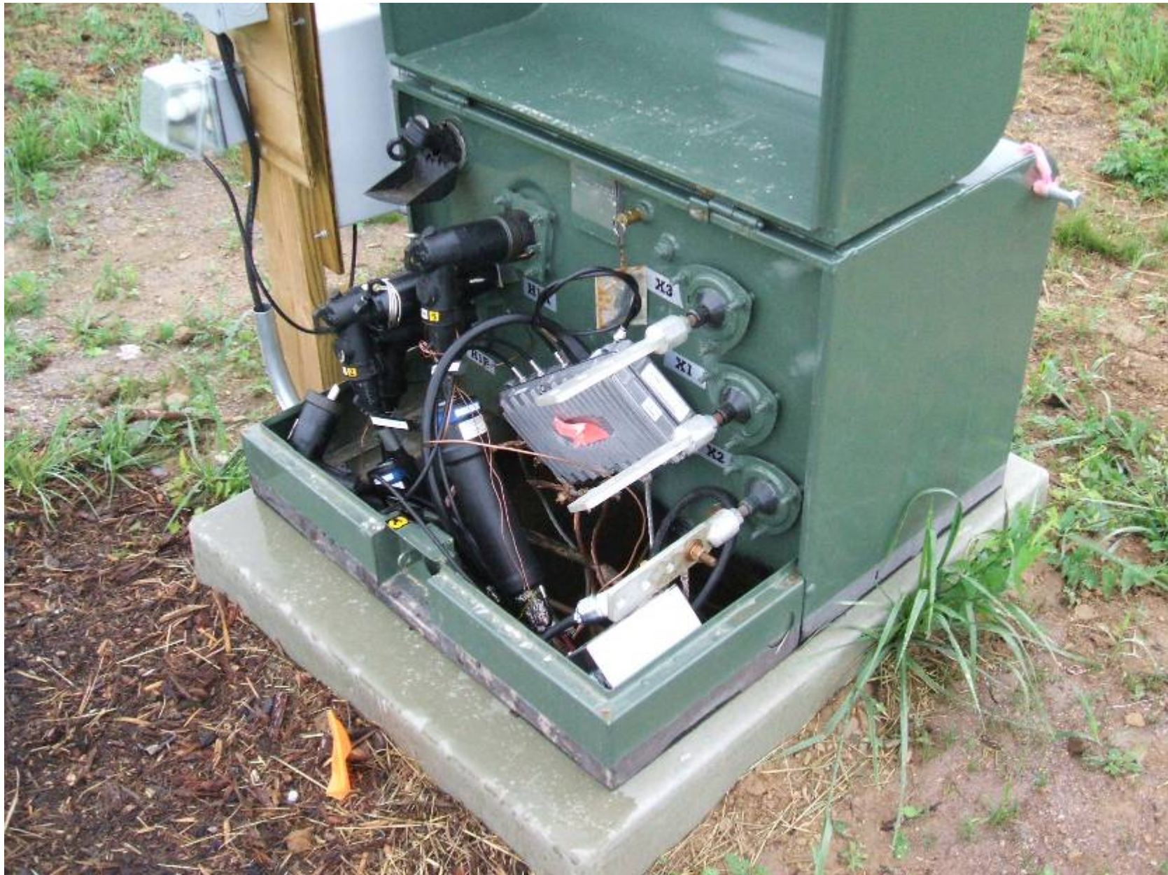
Photograph B-10: Test Site Photo – CURRENT Technologies Field Research and Test Area - XFMR X3 - Interior view, MV3 Bridge
