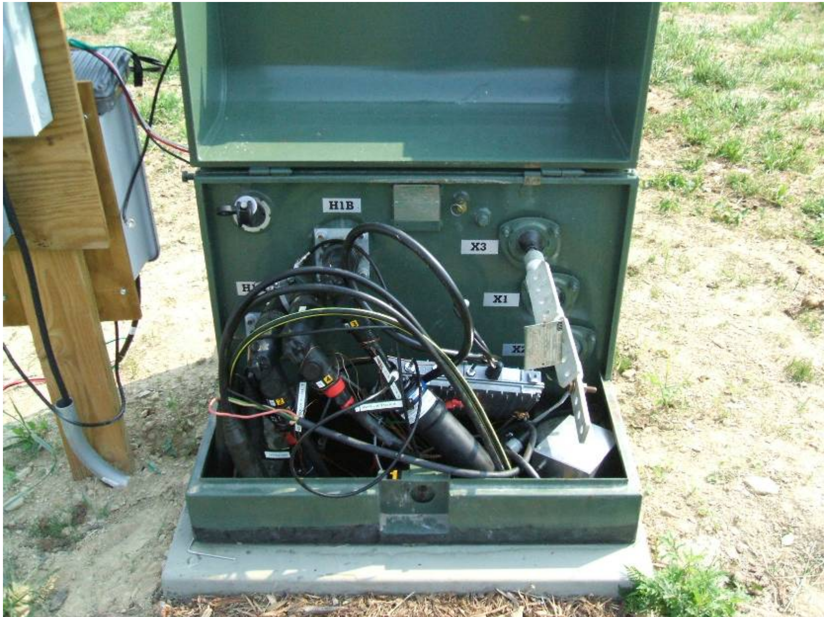
Photograph B-6: Test Site Photo – CURRENT Technologies Field Research and Test Area - XFMR X1 - Interior view, MV3 Bridge
