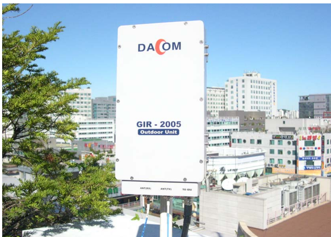
Fig. 3-3 GIR-2005 ODU Installation
