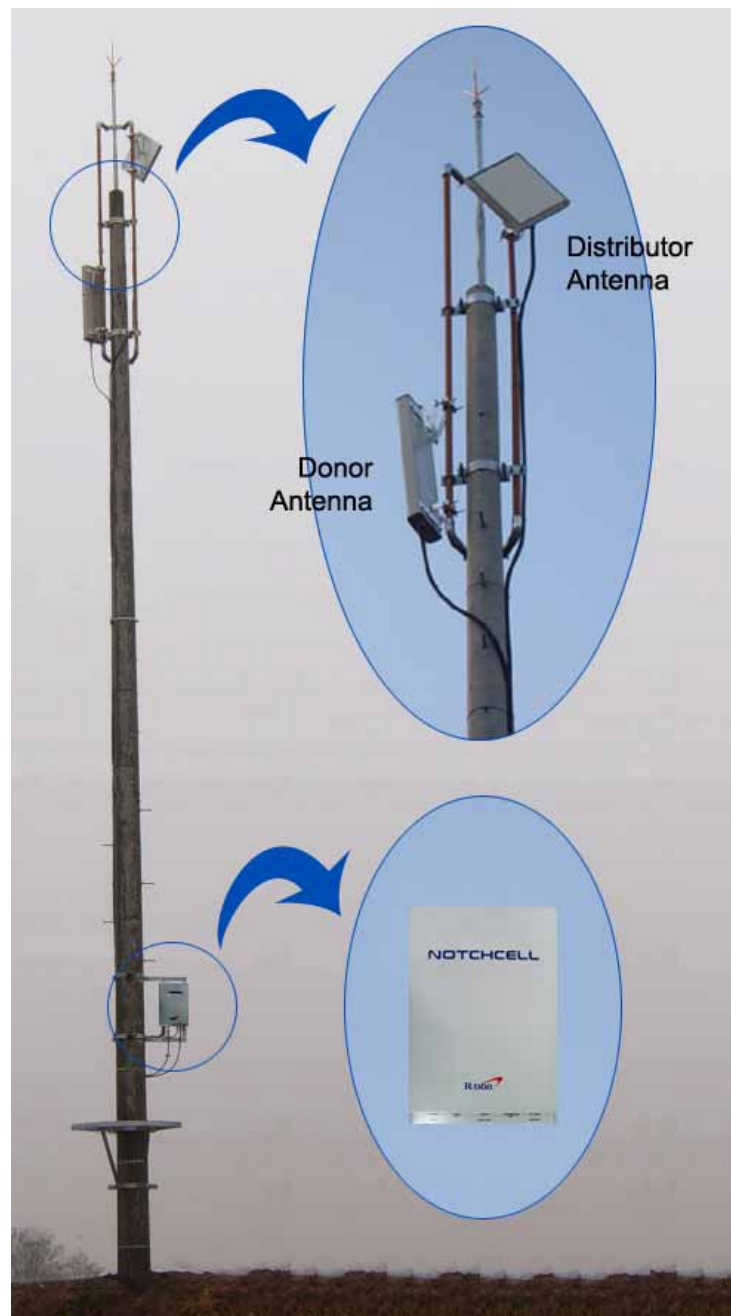
Figure 4.1 Repeater Installation (electric pole type)
