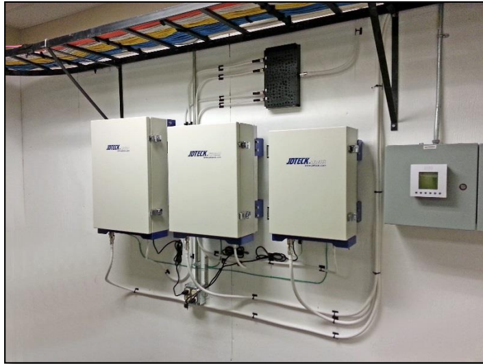
Example of repeaters installed in communications closet.
