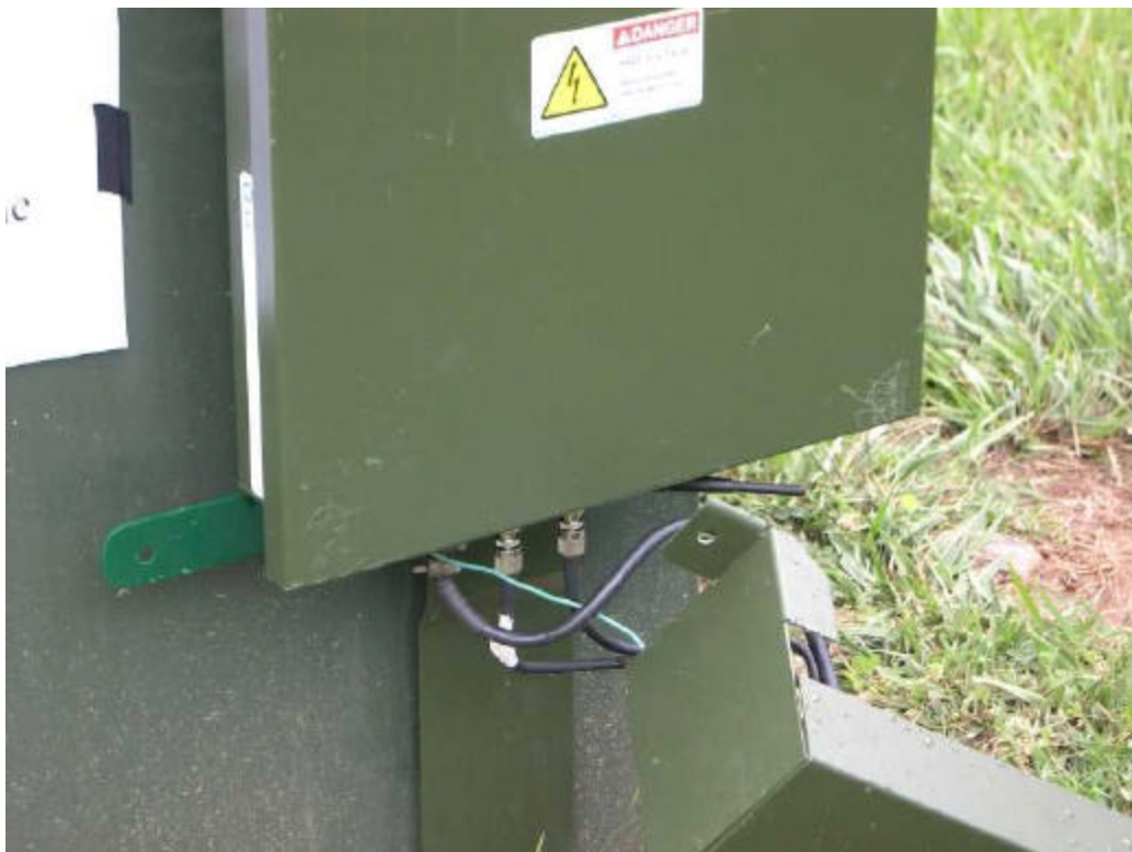
Installation detail showing modem connections to cable couplers
