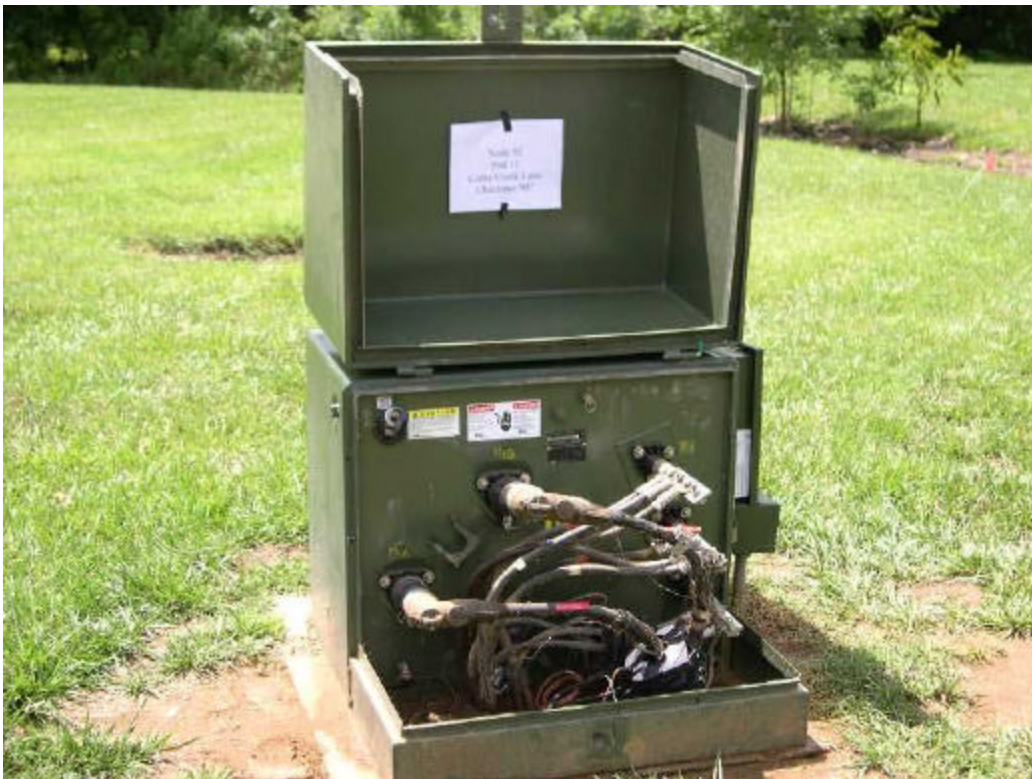
Installation of inductive underground couplers on the MV and LV cables
