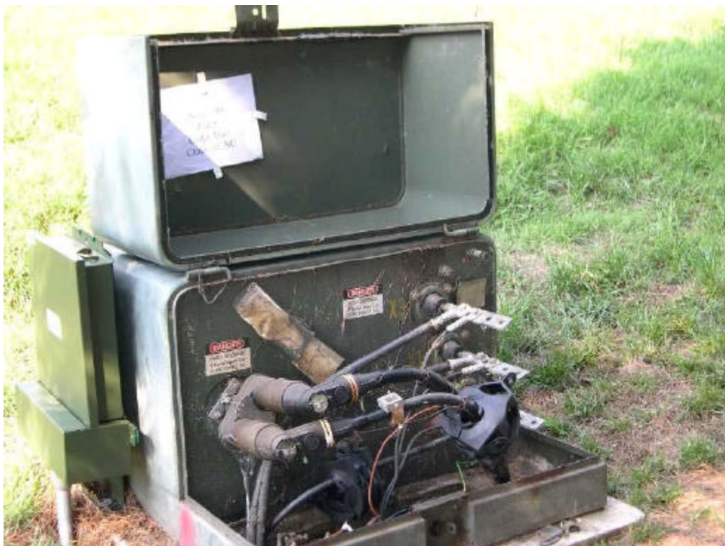
Installation of the inductive underground couplers on the MV and LV cables
