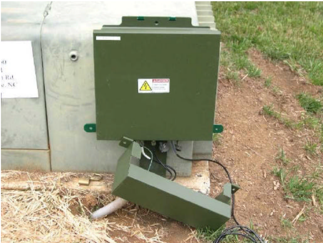
Installation of the inductive underground coupler on MV and LV cables
