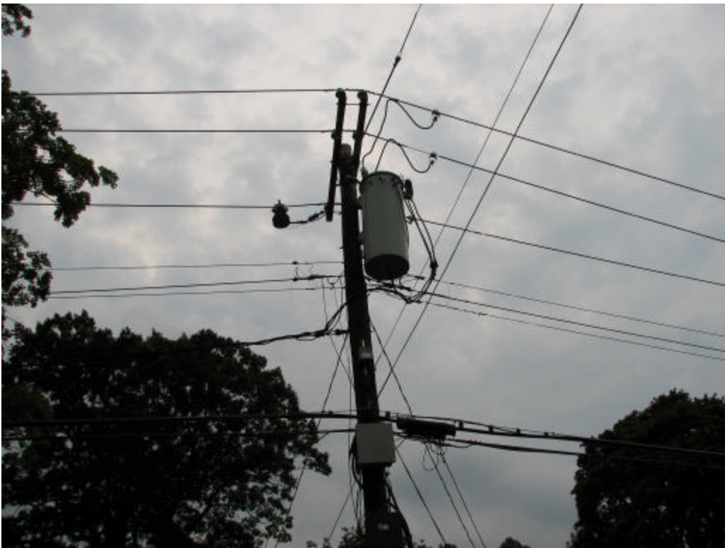
Installation of the overhead MV inductive coupler on the MV line and LV capacitive coupler on the LV line
