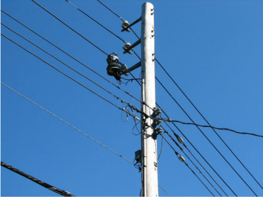
Installation of the overhead MV inductive coupler on the MV line
