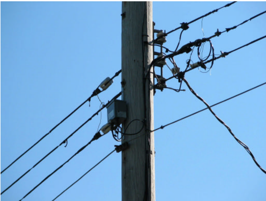
Installation of the LV capacitive coupler on the LV line
