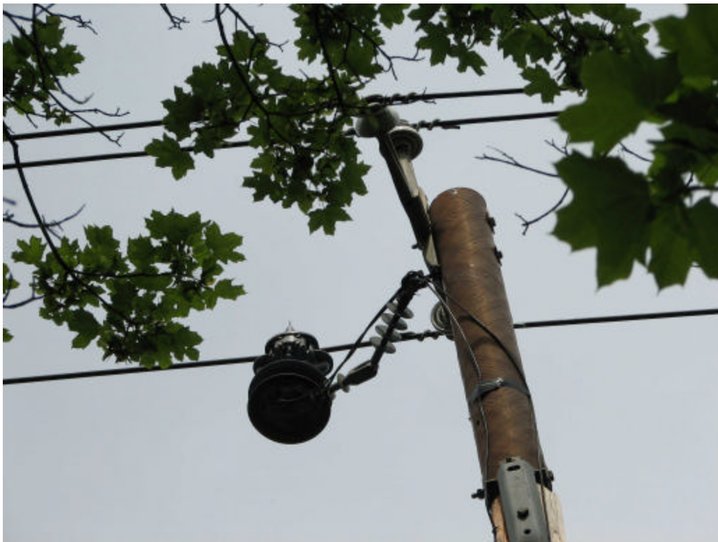
Installation of the inductive overhead MV coupler on the MV line
