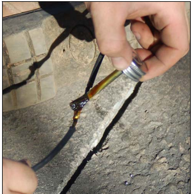
Applying ScotchKote sealer
