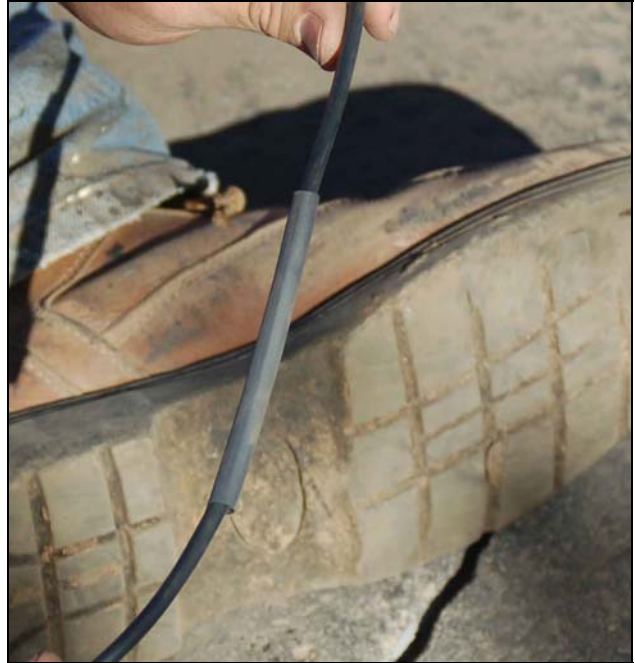
Splice before heating the shrink tube
