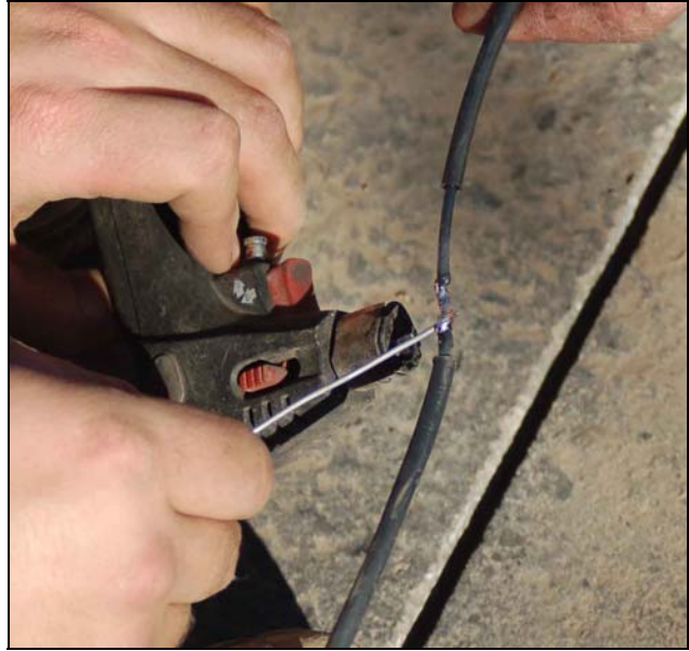
Soldering the splice
