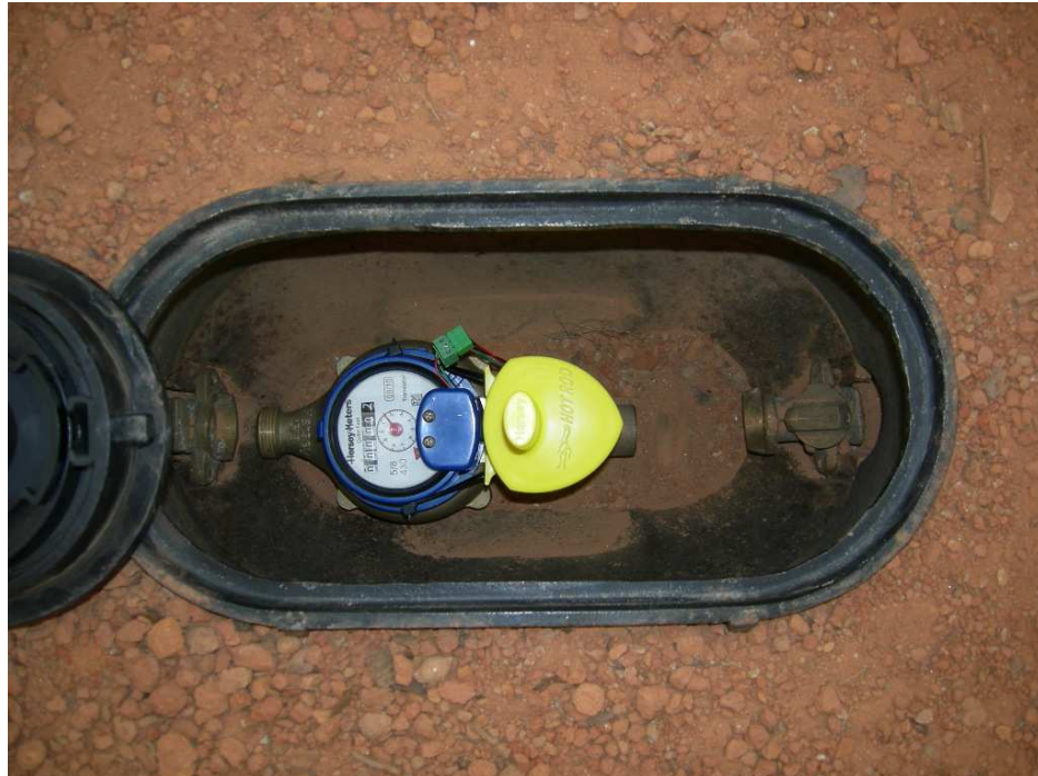
Figure 1: Radiated Emissions – Metal Pit with Composite Lid
