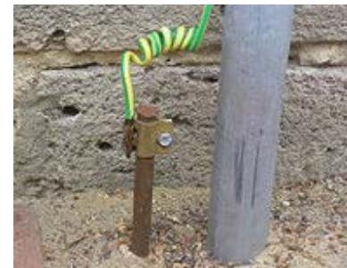
The mechanical installation must ensure that the Array is grounded to earth ground to dissipate static electric charge that may develop due to wind. In Step 3, you secured a grounding wire to the Array (see Step 3 if this has not been done).
