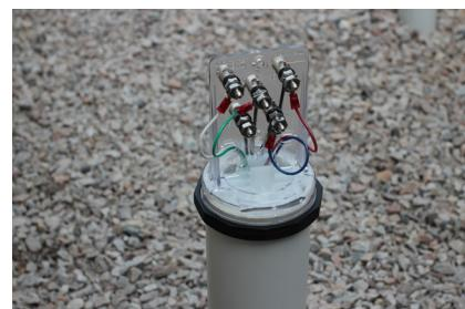
8. Before inserting the CP Test Point, carefully guide and push back all wires back down into the riser.
