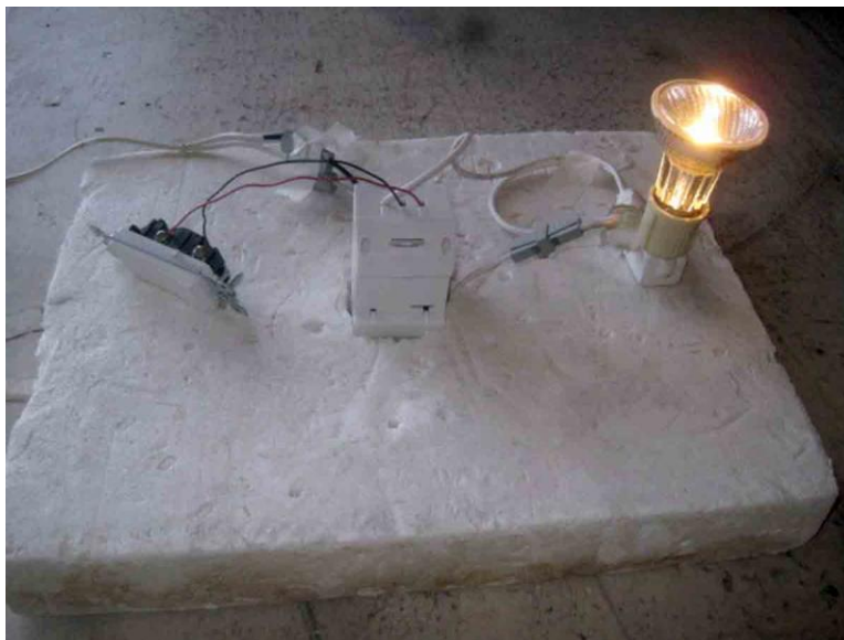
DIMMER & RELAY, BACK VIEW
