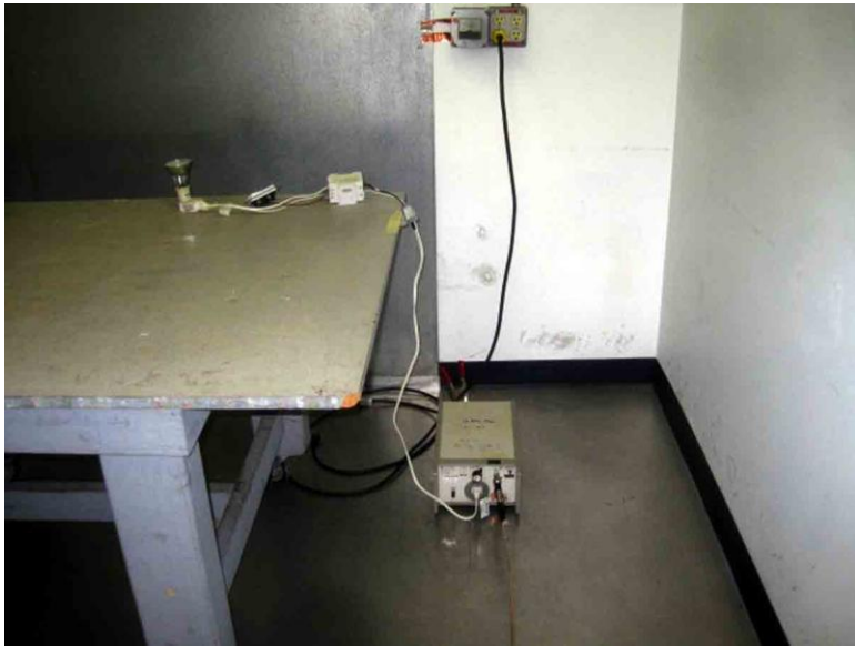
DIMMER, LIGHT OFF
