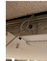
FIGURE 3 Attaching the Cable to a Structurally Sound Anchor
