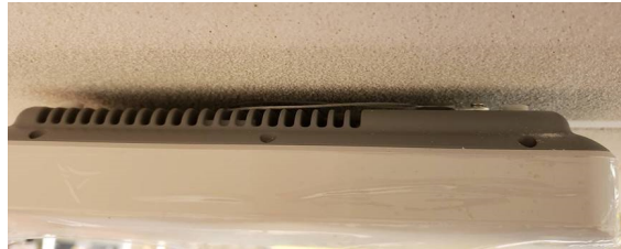
FIGURE 6 Tucking Excess Cable
