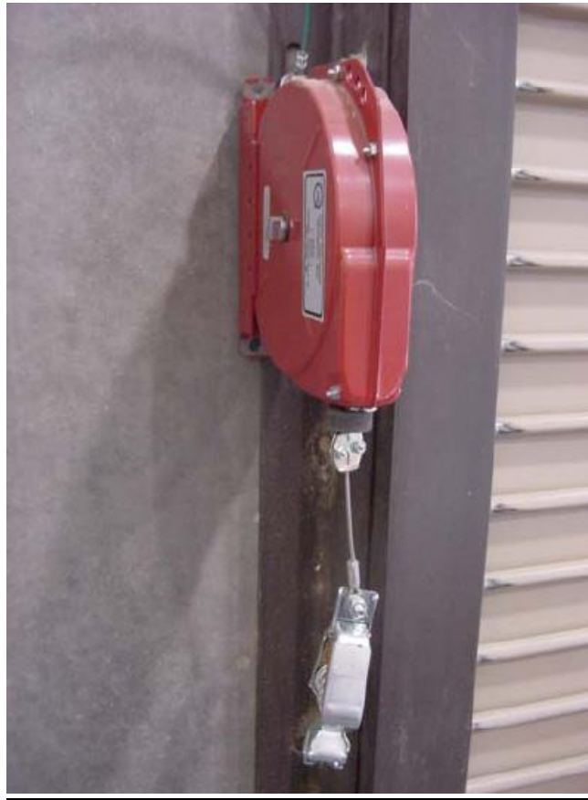
Figure 3.1 – Ground Wire Clip
