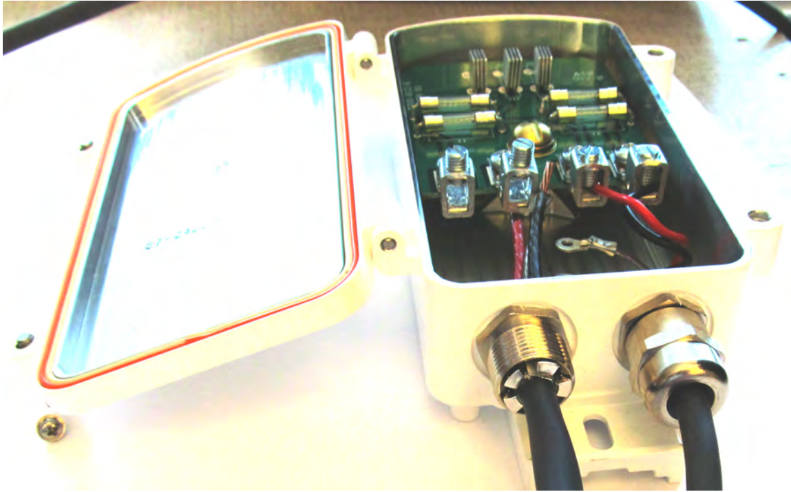
Figure 6-10 Inserting power cable into the LPB
