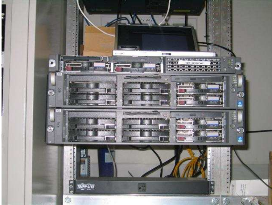
Figure 10: Key Server, BSC and TRAU Servers (top to bottom)
