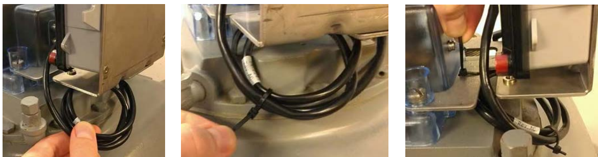
Figure 15 - 6. Coil Excess Cable
