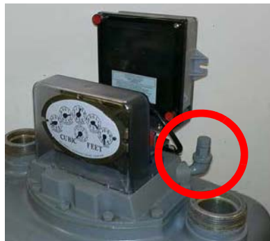
Figure 11 - 1. Meter Pressure Tap
