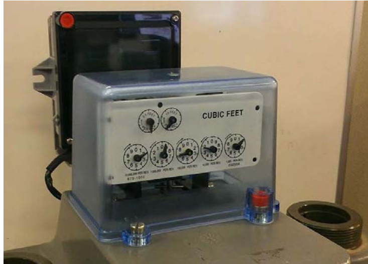
Figure 16 - 7. GPR and Index Cover Assembly Installed On a Schlumberger Large Diaphragm Meter
