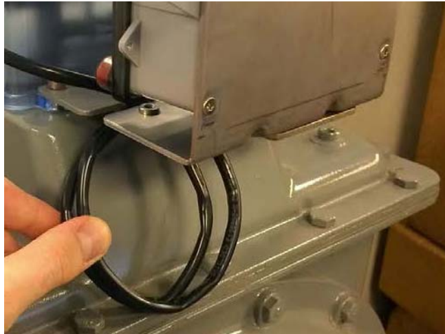
Figure 16 - 5. Coil the Excess Cable
