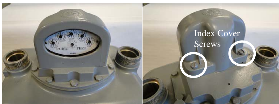
Figure 3 - 1. Rockwell Large Diaphragm Meter Index Cover Front And Rear Views
