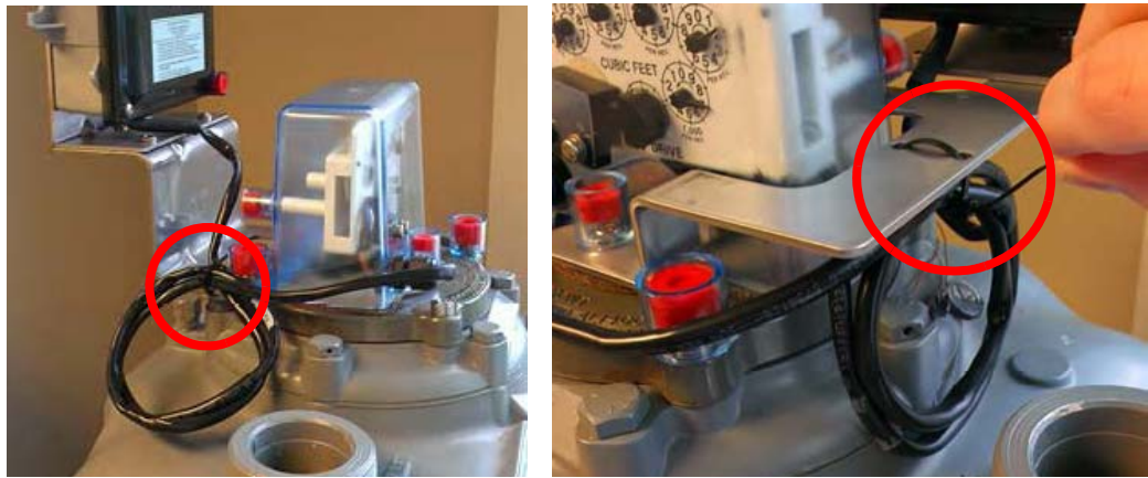
Figure 14 - 6. Left: Coiled Cable Attached to 28-1441 Bracket with Zip Tie. Right: Coiled Cable Attached to 28-1440 Bracket.
