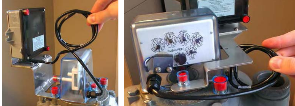
Figure 14 - 5. Left: 28-1441 Bracket. Right: 28-1440 Bracket
