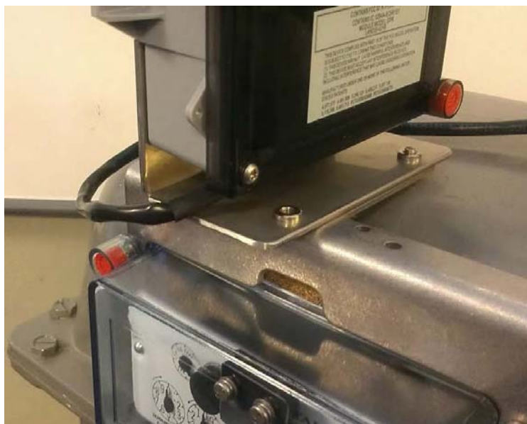
Figure D - 6. Do Not Route the Cable In Front of the GPR Bracket - Route the Cable As Shown in Figure D - 5
