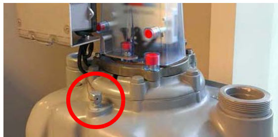
Figure 10 - 1. Installed GPR MUST NOT Interfere with or Block the Pressure Tap
