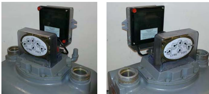
Figure 15 - 9. GPR and Index Cover Installed in Both Orientations
