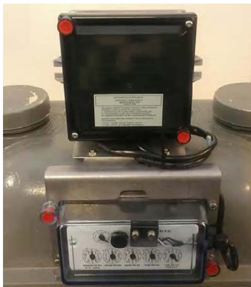
Figure 17 - 7. Switch Wires Must Not Interfere With Index Pointers
