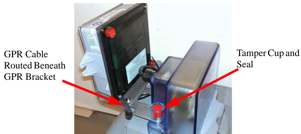
Figure 15 - 7. Install a Seal In Each Tamper Cup
