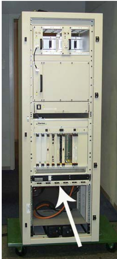
Figure 8.1 Distribution Panel with Circuit Breakers — Front View
