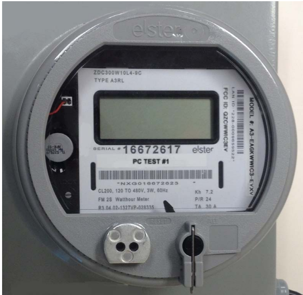
EA_Gatekeeper completed assembly
