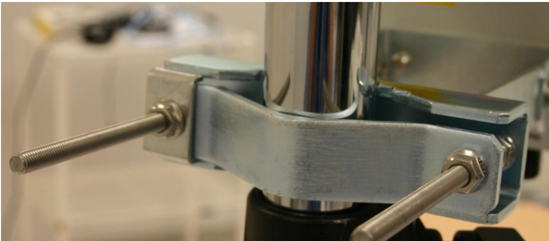
Figure 86 Attaching the AP antenna lower bracket to the pole
