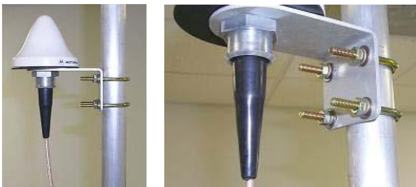
Figure 36 GPS antenna mounting
