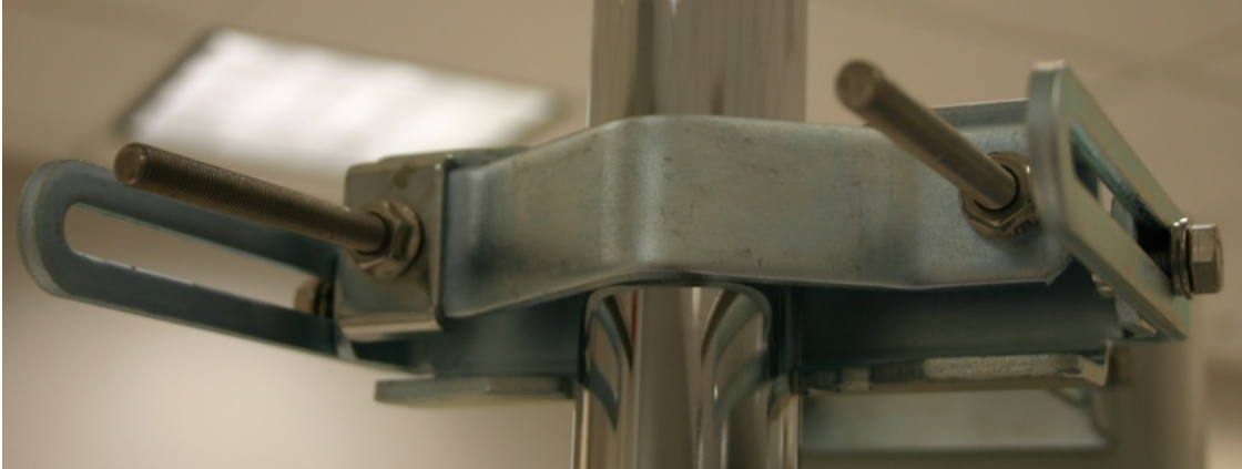
Figure 104 Attaching the AP antenna upper bracket to the pole
