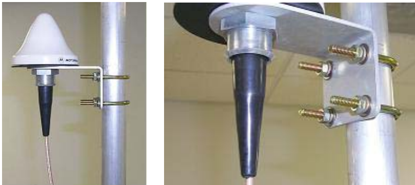
Figure 45 GPS antenna mounting
