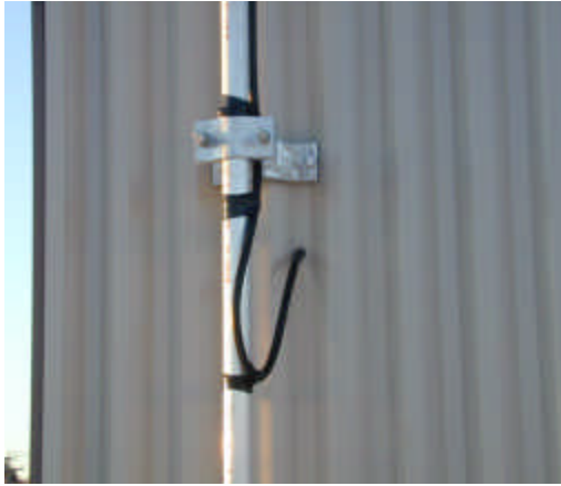
Figure 3-14 Drip loop on the antenna cable.
