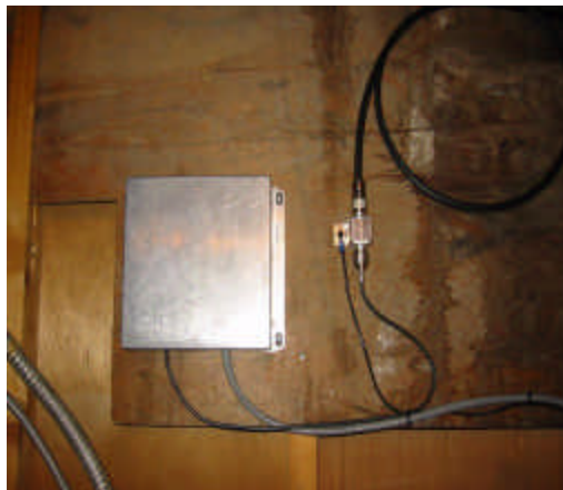
Figure 3-15 Access Point typical installation with surge protector.
