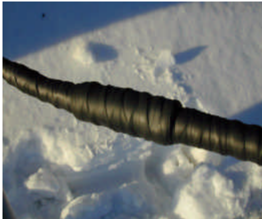
Figure 3-13 Waterproof tape around antenna and the transision coax cable connectors
