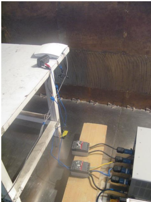
Conducted emissions of AC power port
