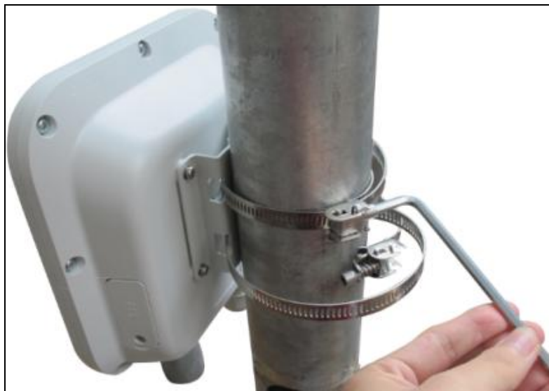
Figure 3-5 Adjusting the length of the hose clamp
