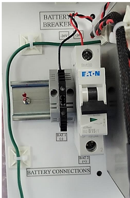
Figure 9: Battery Connections (Pre-Wiring)
