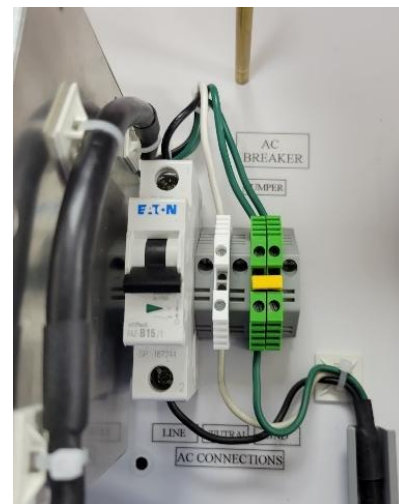
Figure 8: AC Connections (Post-Wiring)
