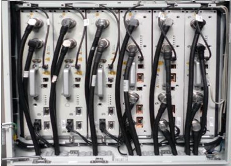
The RF jumpers go out from the base, as shown in [Figure 5-17](#). The cables between cabinets must be protected with protective tubes, without any exposed part of the cables and the openings at two ends of these cables must be sealed, as shown in [Figure 5-18](#).
