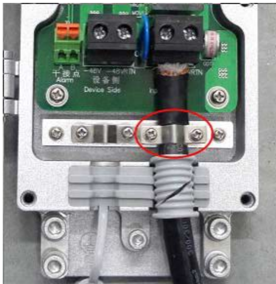
Figure 4-38 PIMDC Connection (to Lightning Protection Box)
